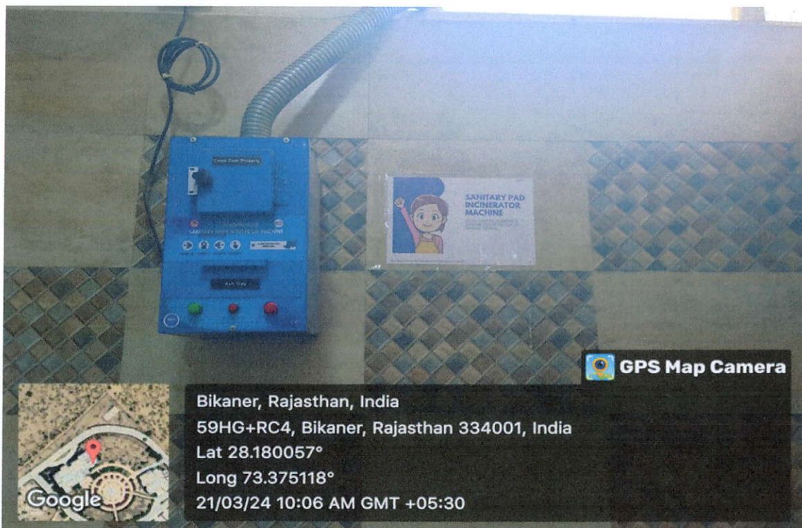
Incinerator for Destroying Biomedical Waste (Used Sanitary Pads)
