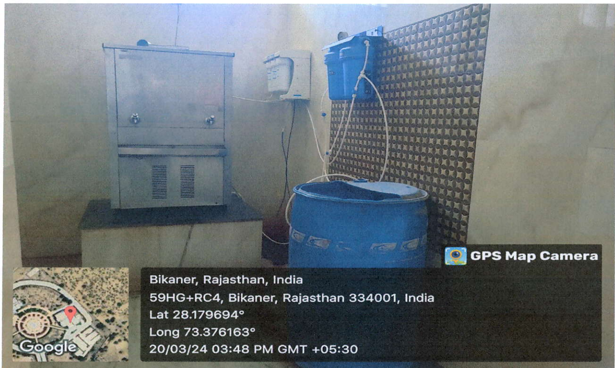
Water Waste from RO is Collected in Drums and Used for Floor Cleaning
