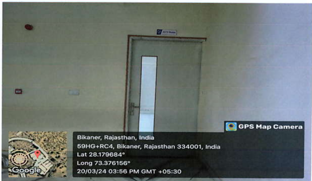
CCTV Surveillance in Campus
