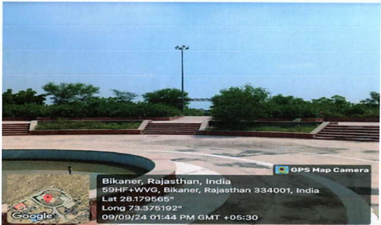
High Mast Lights Installed for Proper Illumination
