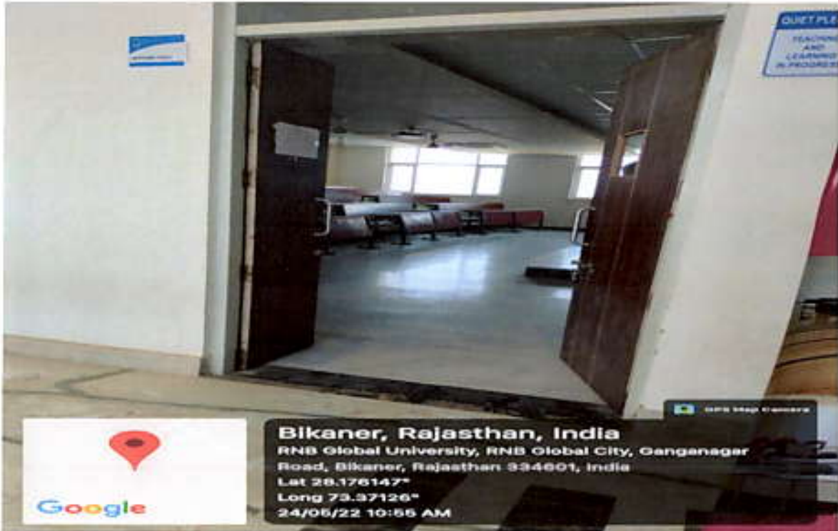
Second Floor Room No. - 214 Classroom front
