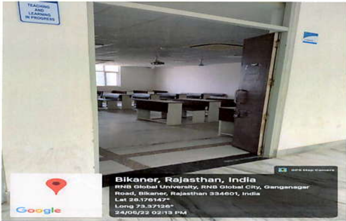
Second Floor Room No. – 202 Classroom front
