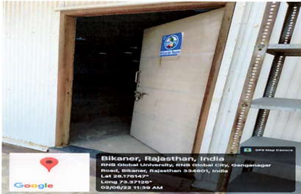
Billiards Room- Front
