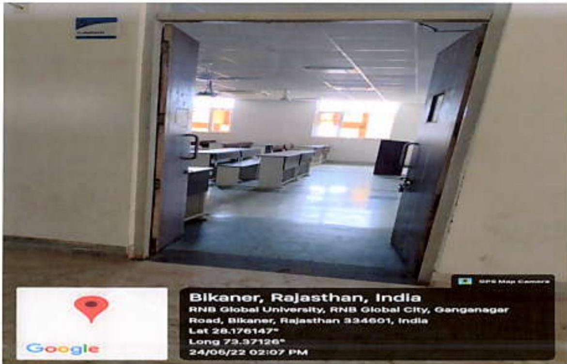
Second Floor Room No. - 212 Classroom front
