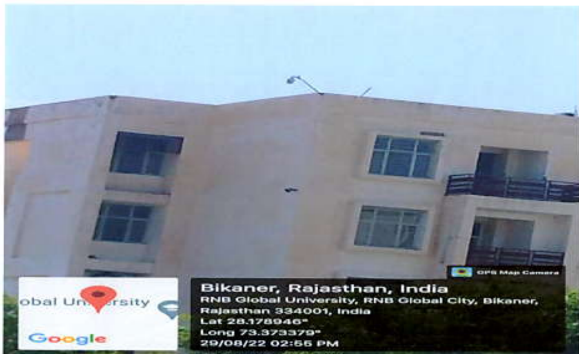
Boys Hostel- CCTV Camera
