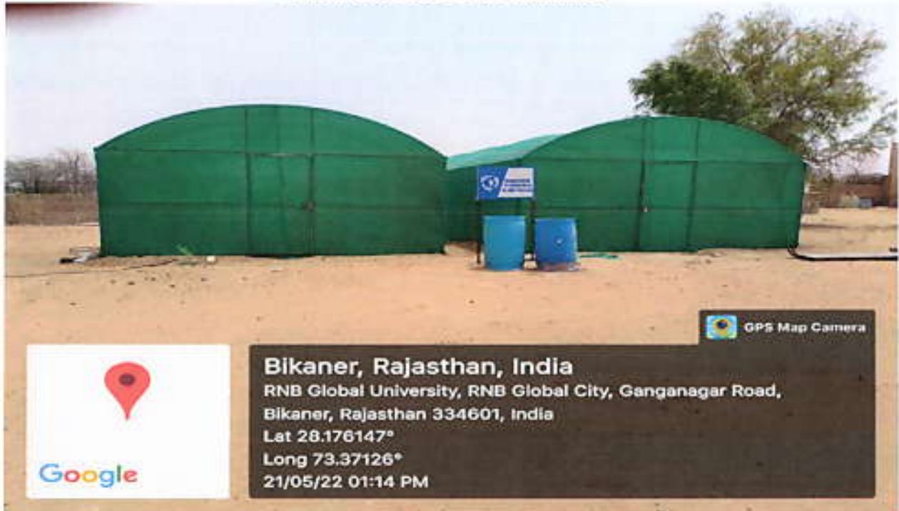
Vegetable Production in Net House- Outside View
