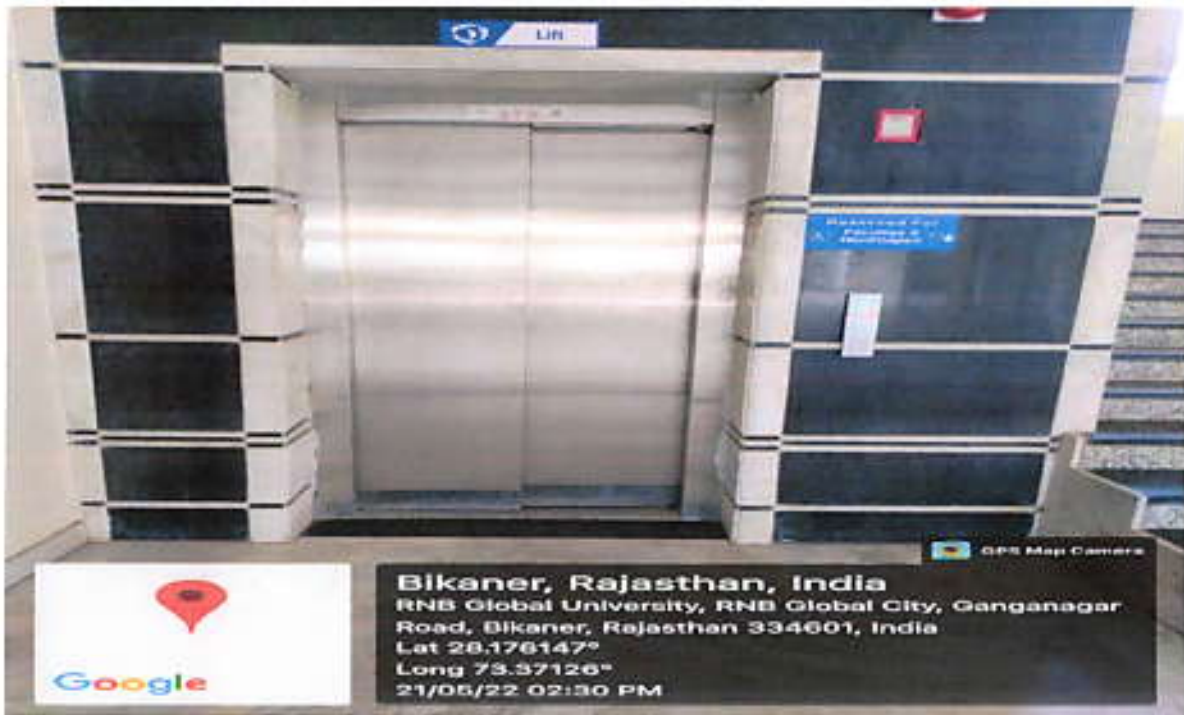
Lift- Administrative block
